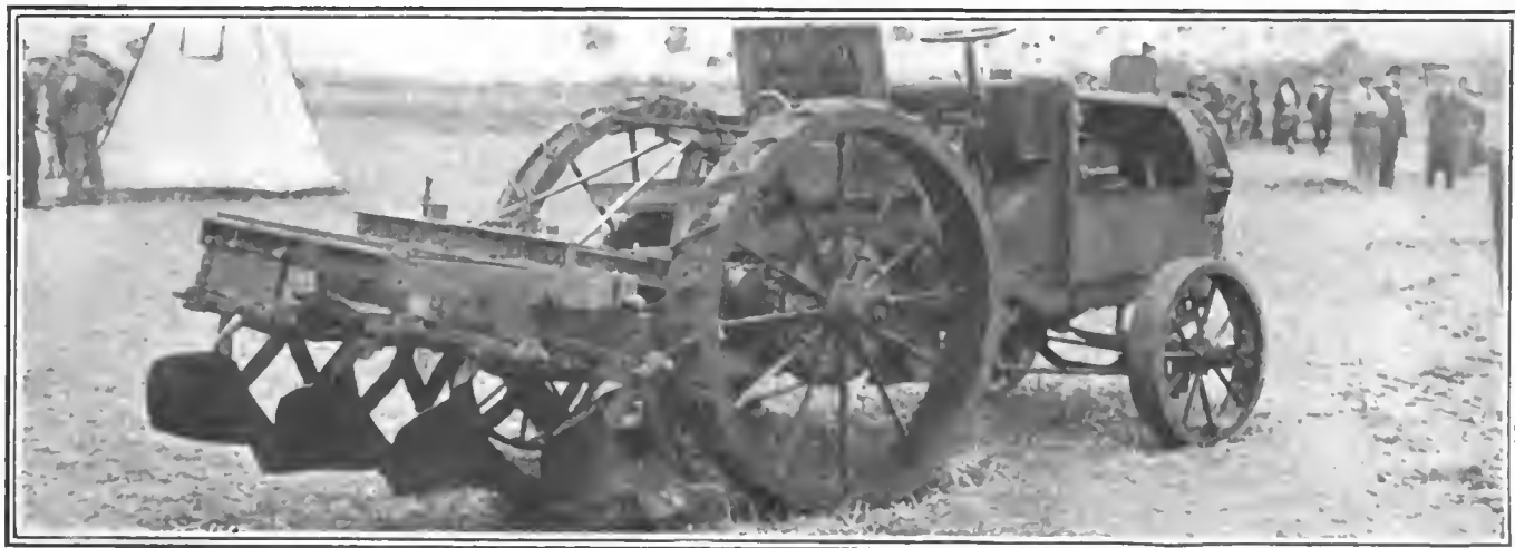
Fig. 4—The Linard-Hubert tractor with its detachable ploughing equipment
